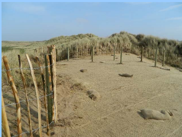
The picture shows an example of working with natural processes by raising the level and reinforcing the natural coastal sand dune system which will ultimately protect the village of Talacre.
